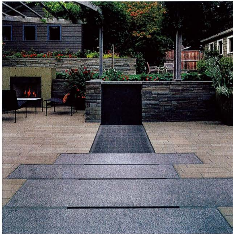
A sleek granite waterfall is set into the bluestone retaining wall. Concrete slabs and grating cross the water runnel so that 100 percent of the patio space is usable.
